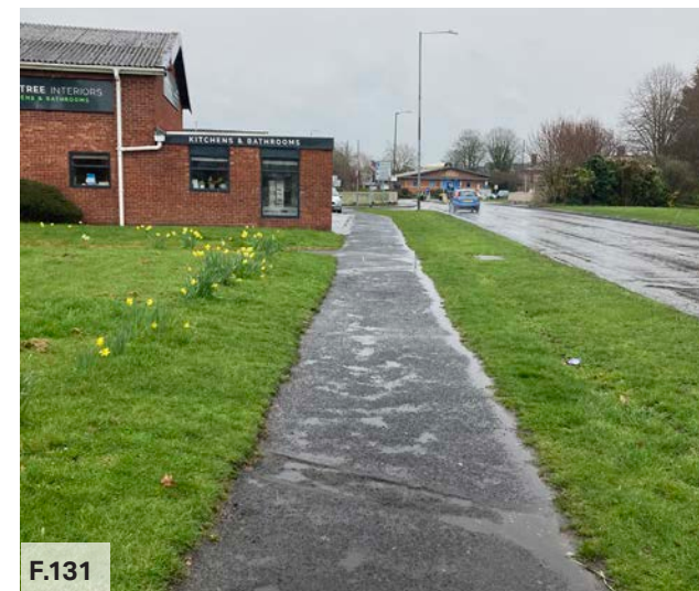
Figure 131: Footpath on Ombersley Way
